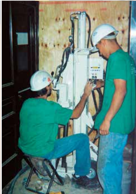
Collecting geotechnical samples for a new elevator shaft.
